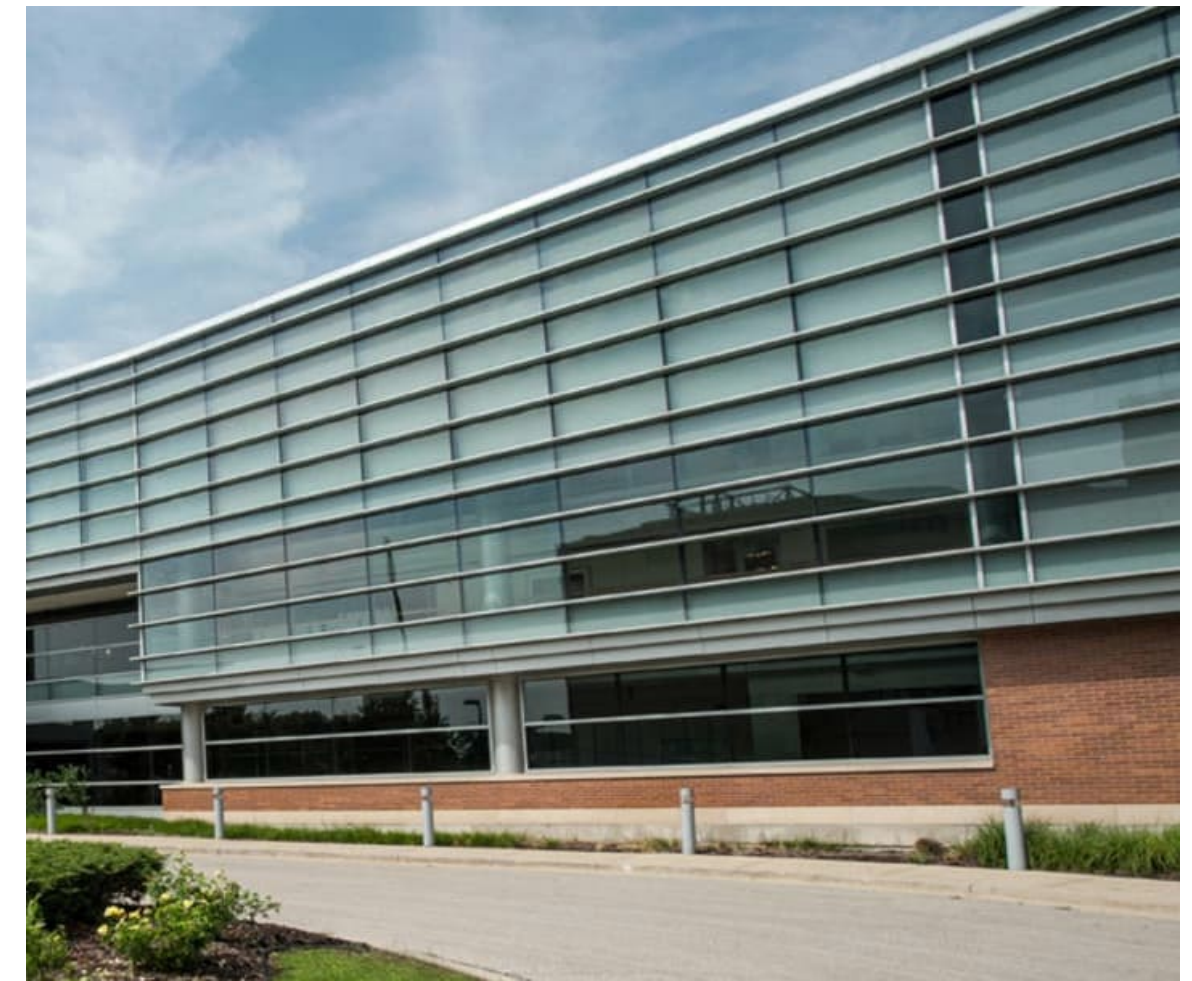
Curtain wall façade with horizontal metal sunscreen
